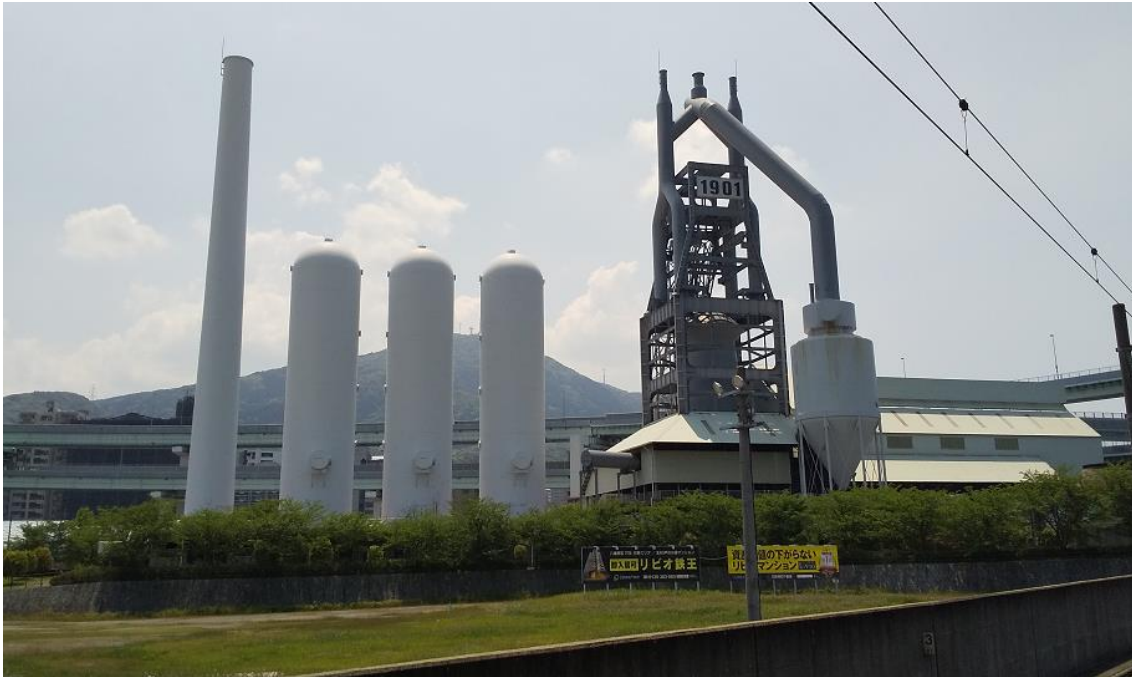
Fig. 2. Higashida First Blast Furnace as the core of Yawata steel works established in 1901 in Yahata-higashi ward, Kitakyushu symbolizes the industrial revolution in Asia.
