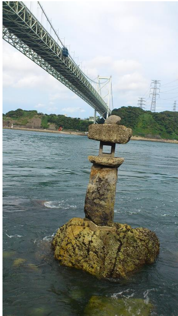
Fig. 4. The Kanmon bridge across the Kanmon channel and the stone lantern belonging to Mekari shrine (viewed from Kyushu side). At that time of construction, the Kanmon bridge was the longest suspension bridge in Asia.
